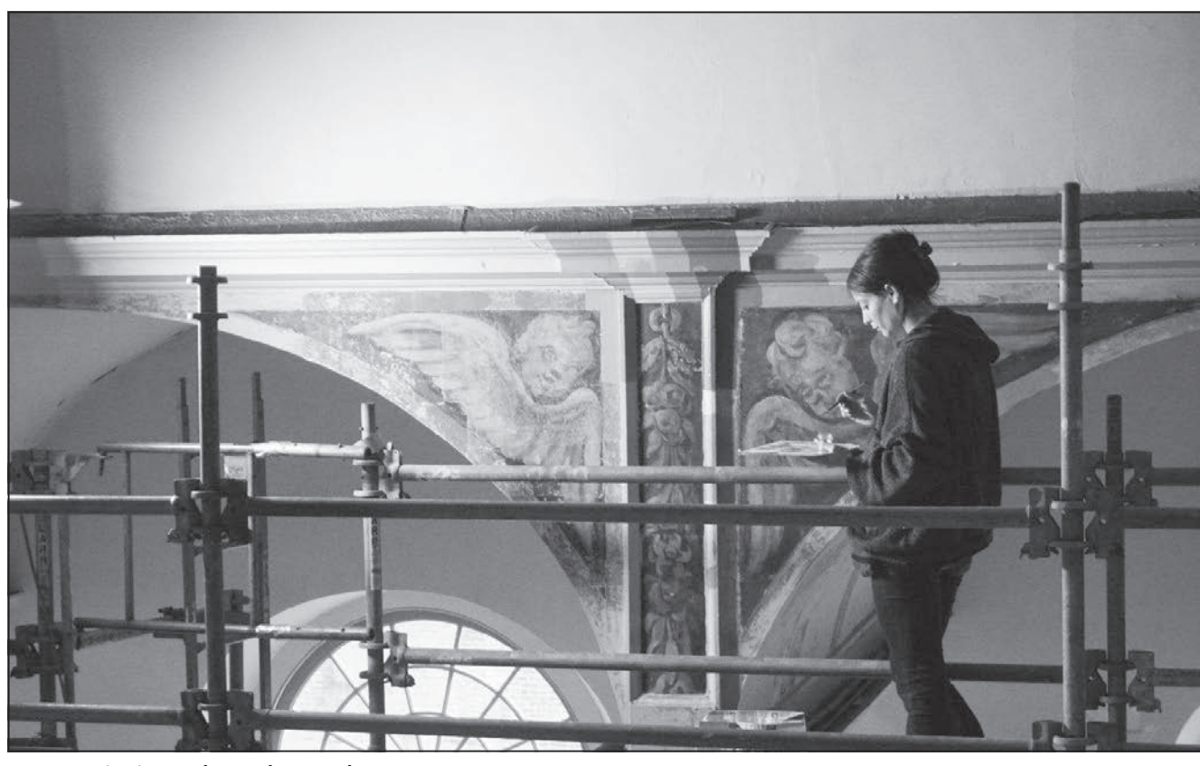
A restorationist works on the angels.
