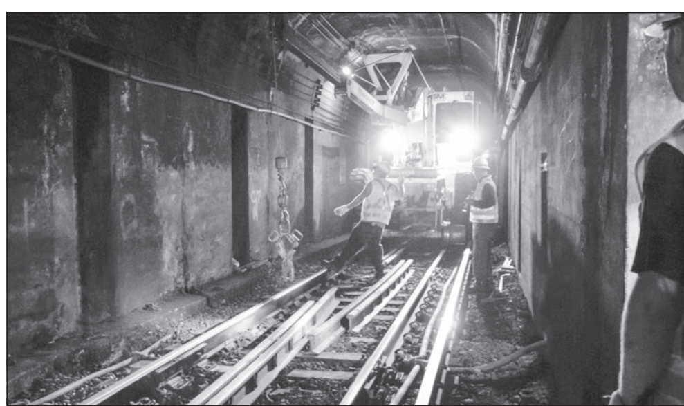
The MBTA will close the Blue Line from Airport to Bowdoin for nearly two weeks next month for tunnel repair work.
