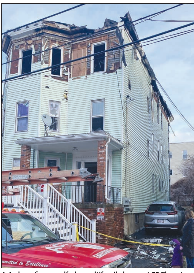
A 4-alarm fire engulfed a multifamily home at 53 Thornton St., early Tuesday morning, displacing 19 people, and costing one resident their life.
