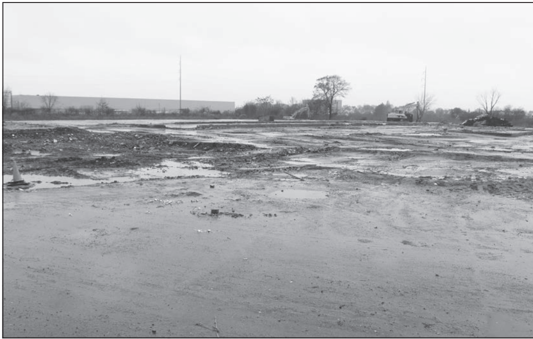
The site of the former Wonderland Greyhound Park stands bare following the building's demolition.
